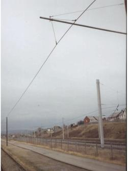
We also hold patents for our OHL, which is simple and quick to install. It is suitable up to 160km/h. In the background of the photograph are the West Coast Mainline (WCML) gantries and overhead (at Carnforth, England).
